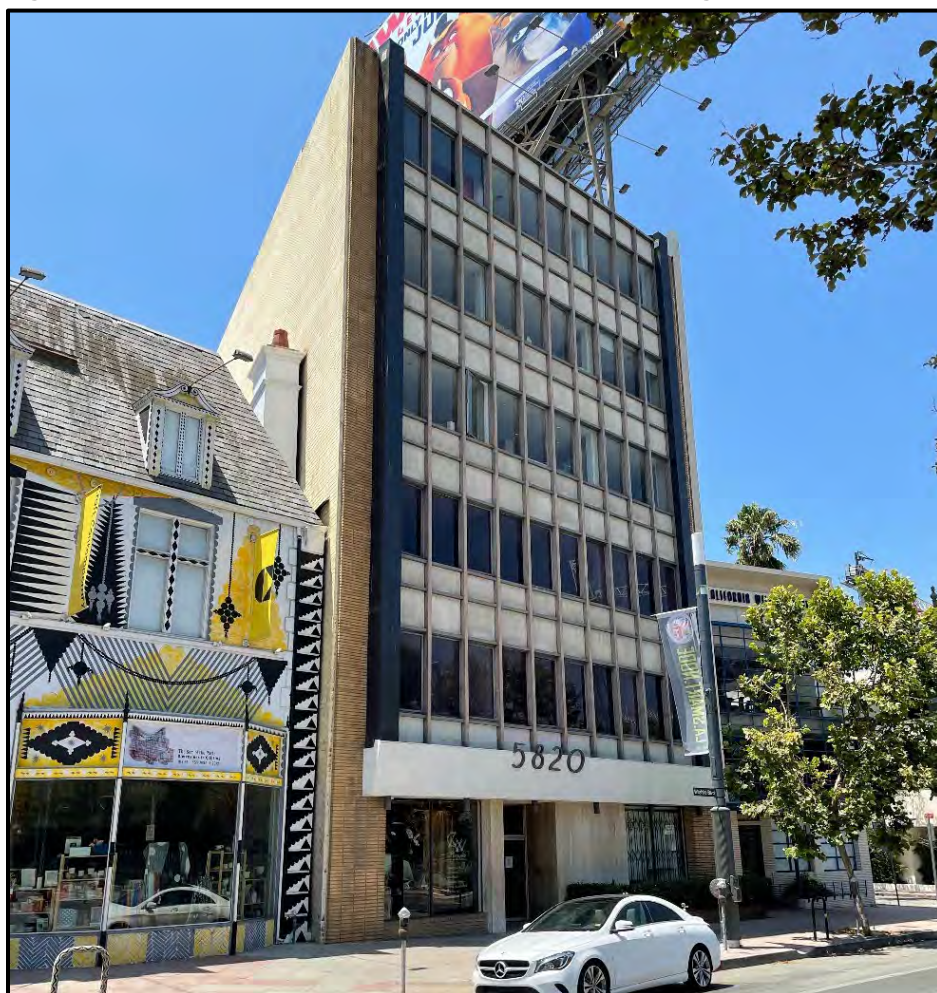
Figure 74. 5820 W. Wilshire Boulevard, Hancock Park Building
