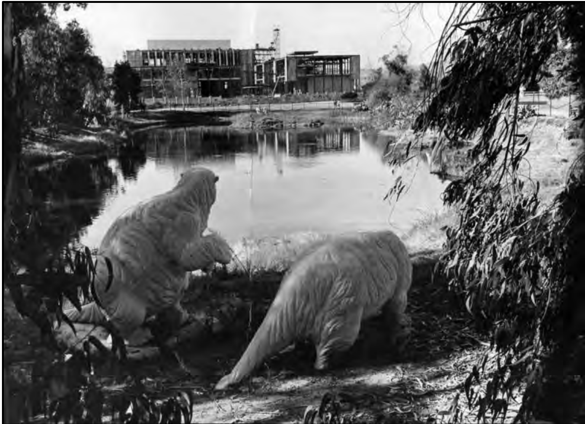
Figure 38. LACMA under construction in 1964, view facing west across Lake Pit (top) and 1964 aerial showing LACMA in western portion of Hancock Park
