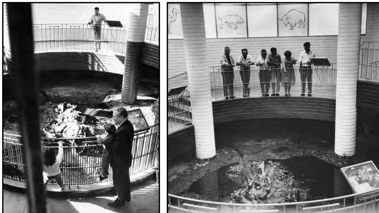
Figure 44. Interior of the Observation Pit, 1964 (left) and 1967 (right)
