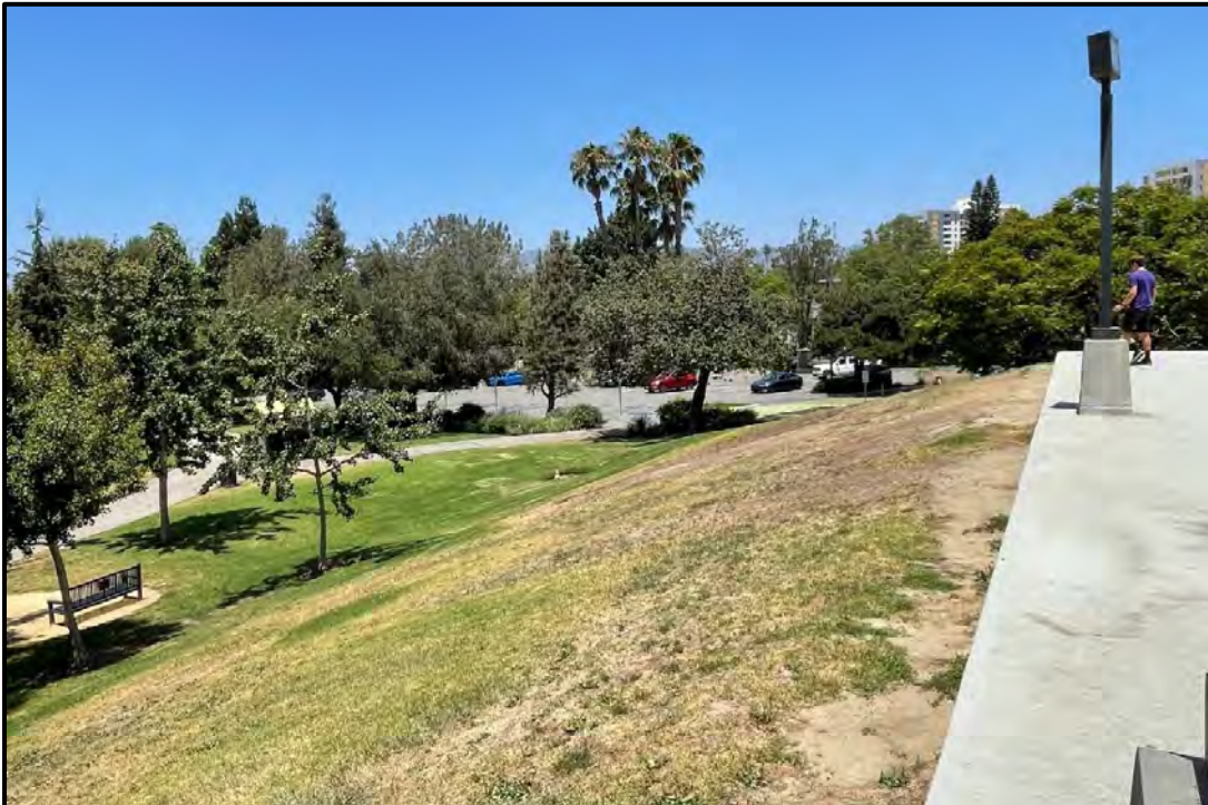
Figure 63. Page Museum podium and berm, west elevation
