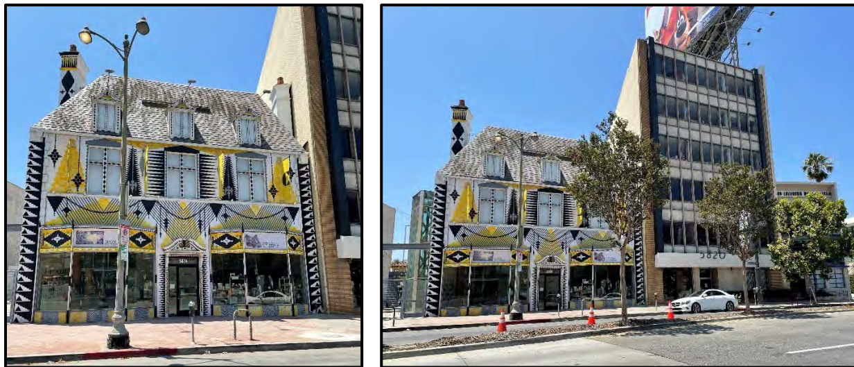
Figure 73. 5814 W. Wilshire Boulevard, Craft and Folk Art Museum, detail (top) and context (bottom)
