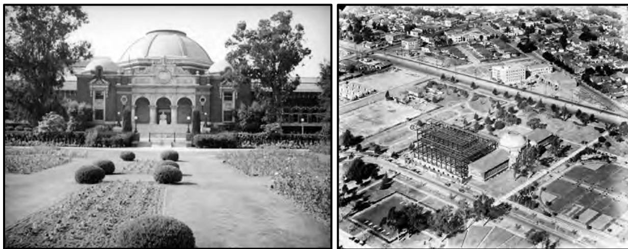
Figure 17. Original 1913 building of the Los Angeles County Museum of History, Science, and Art in Exposition Park, ca. 1930 (left); Los Angeles County Museum of History, Science, and Art, with expansion under construction, ca. 1925 (right)
