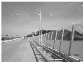
Figure 5.7. Partially shielded noise screens, installed during the construction of a new motorway in the Netherlands for avoiding light trespass to a compensation area with bat habitats (© V. LOEHR).
